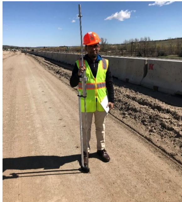
Figure 11. Interstate 25 South Gap Test Site in Larkspur
