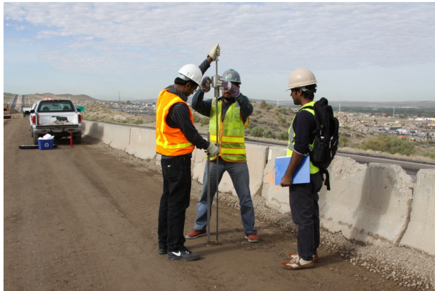
Figure 1. Conduction of DCP on Interstate 25 (I-25) in New Mexico
