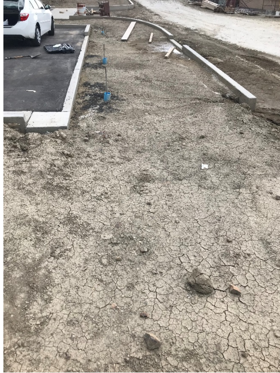
Figure 8. School Parking Lot Test Site in Pueblo, CO.
